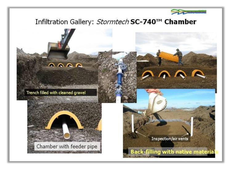
Figure 59. Infiltration Gallery #3 - Stormtech Chamber Installation (2008)
