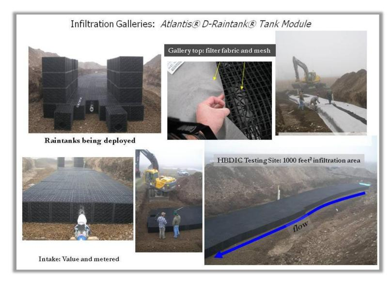
Figure 60. Infiltration Gallery #4 - Atlantis Raintanks Installation (2008)
