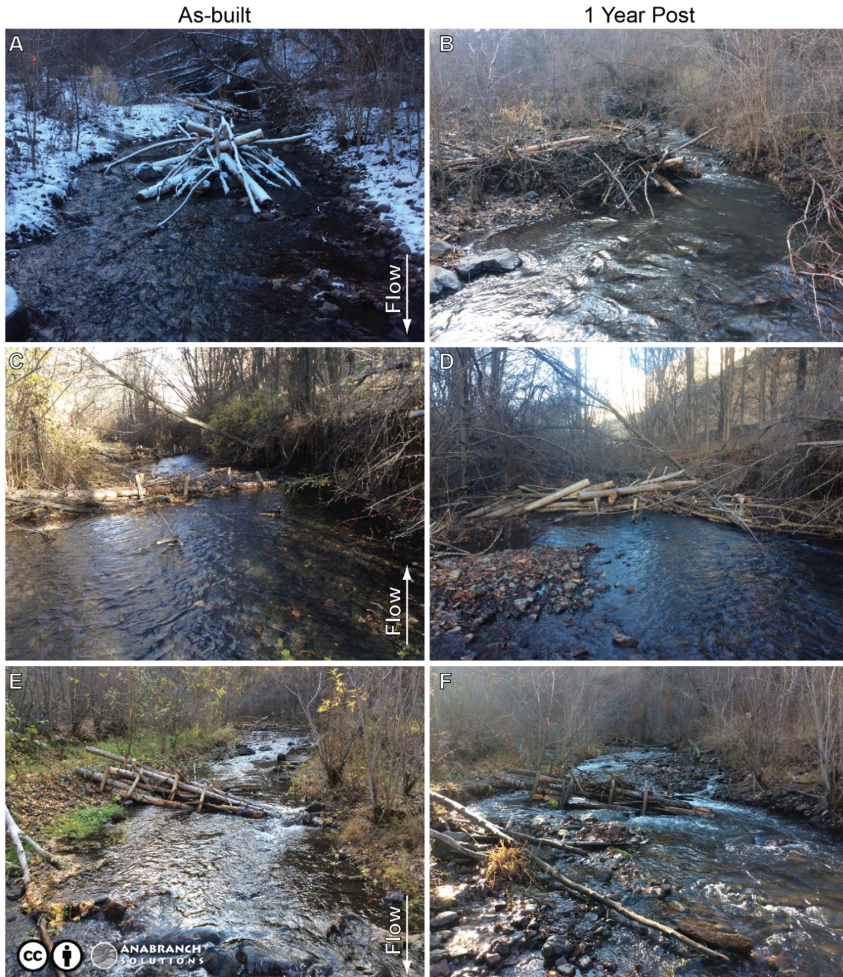
Figure 14: Example of PALS evolution over the course of one year promoting processes of wood accumulation. A and B show a mid-channel PALS becoming a bank-attached PALS, C and D show a bank-attached PALS becoming a debris jam, and E and F show a bank-attached PALS becoming a mid-channel PALS. The geomorphic changes imposed by the presence of the PALS in each example shows clear alterations to the channel bed and hydraulics. From Chapter 4 of Wheaton et al. (2019: http://lowtechpbr.restoration.usu.edu ).
