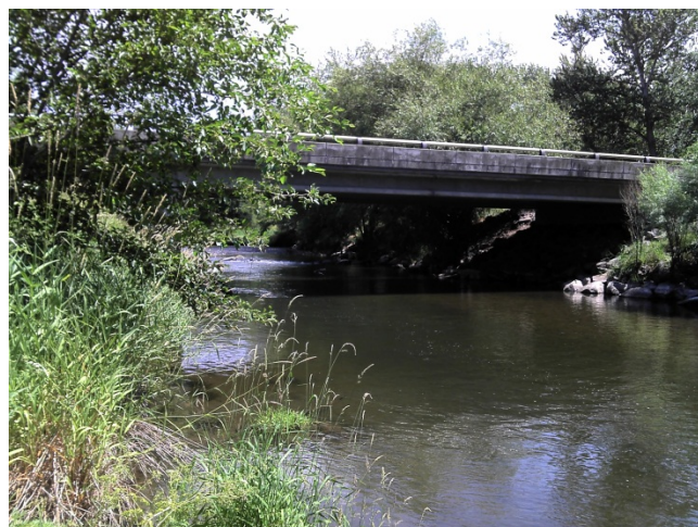
Hart Road Bridge measuring site
