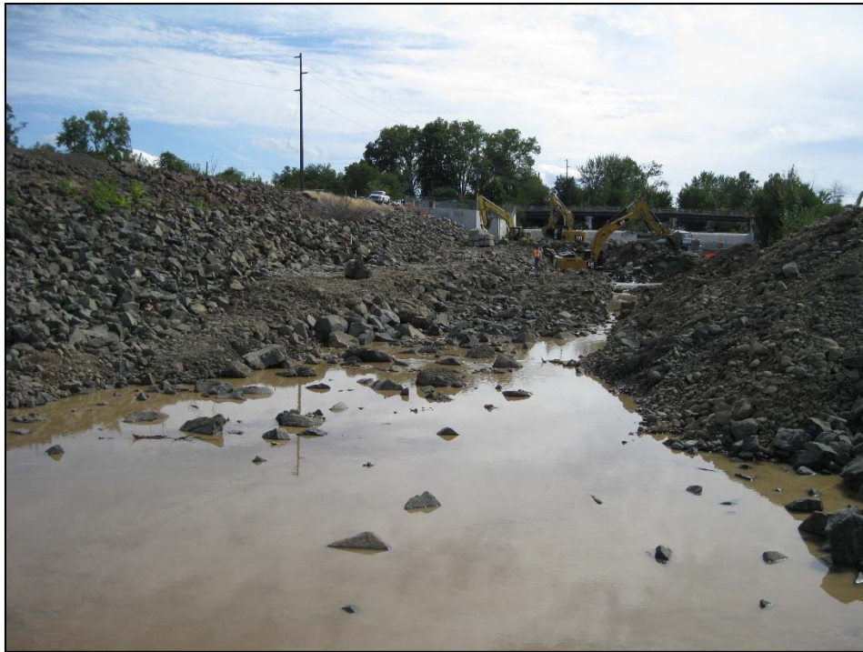
Milton Freewater Levee Section, Walla Walla River, September, 2014
