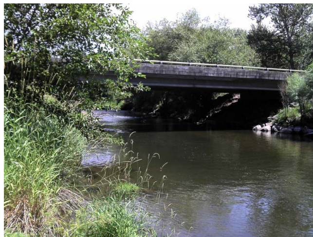
Hart Road Bridge measuring site
