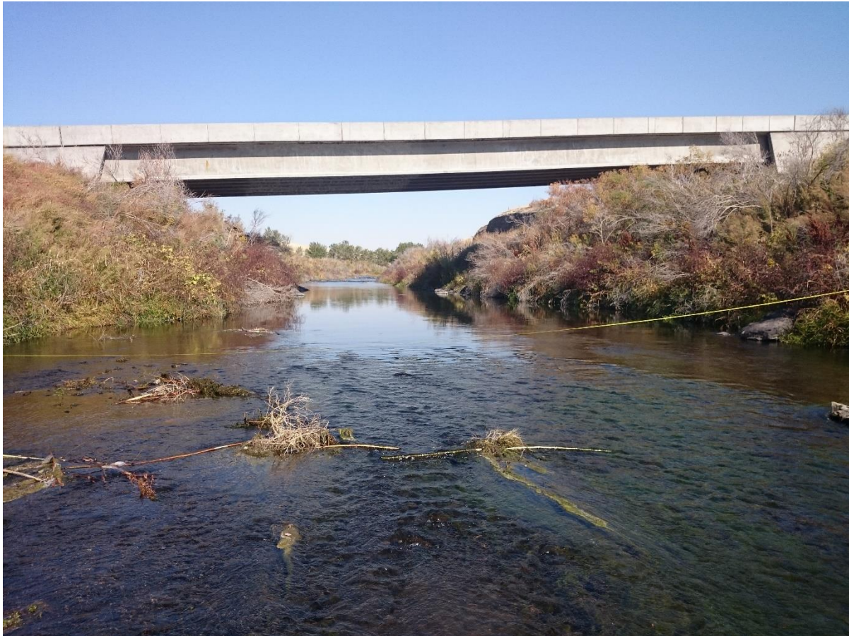
Touchet River at IW Sims Road Bridge
