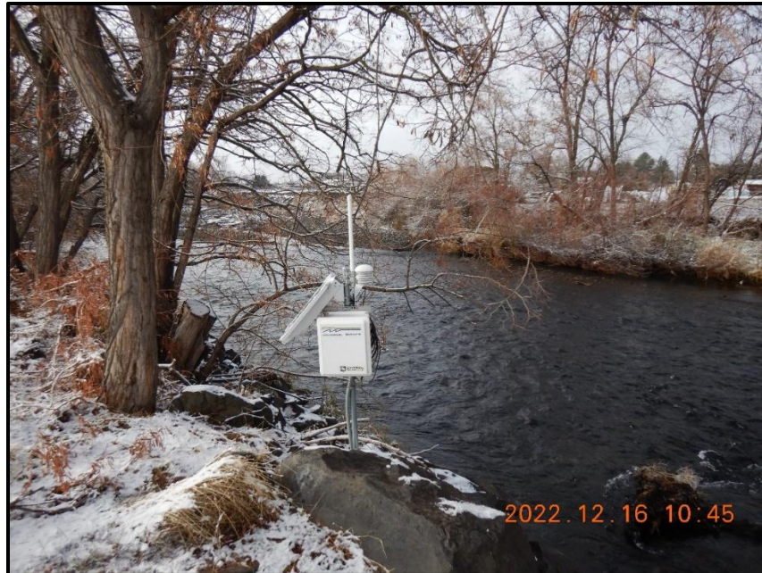
Figure 4. At this near real-time monitoring site on the South Fork Walla Walla River (S-107), a cabled sensor secured to a boulder collects water level data. A communication cable transmits the information to a data logger and radio housed in the gauge box. Using radio telemetry, water level data was sent to the WWBWC office to be processed and published online.
