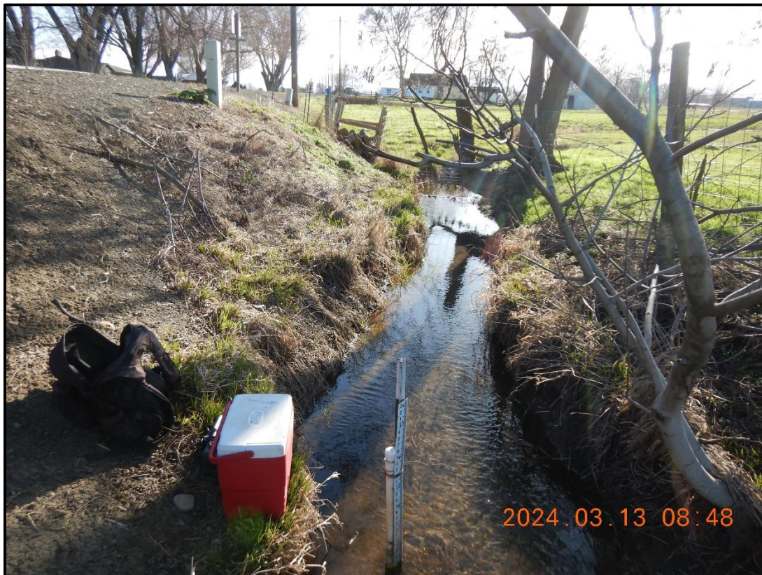
Figure 6. At this stand-alone monitoring site on the West Little Walla Walla River (S-222), a staff gauge and perforated PVC stilling well enclose a suspended pressure transducer.
