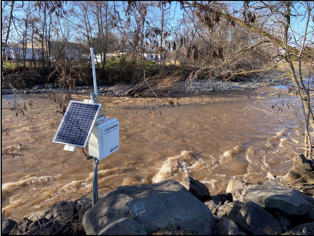
Figure 4. At this near real-time monitoring site on the Walla Walla River (S-107), a cabled sensor, secured to a boulder in the channel, collects water level data. A communication cable transmits the information to a data logger and radio housed in the gauge box. Using radio telemetry, water level and temperature data are sent to the WWBWC office to be processed and published online.
