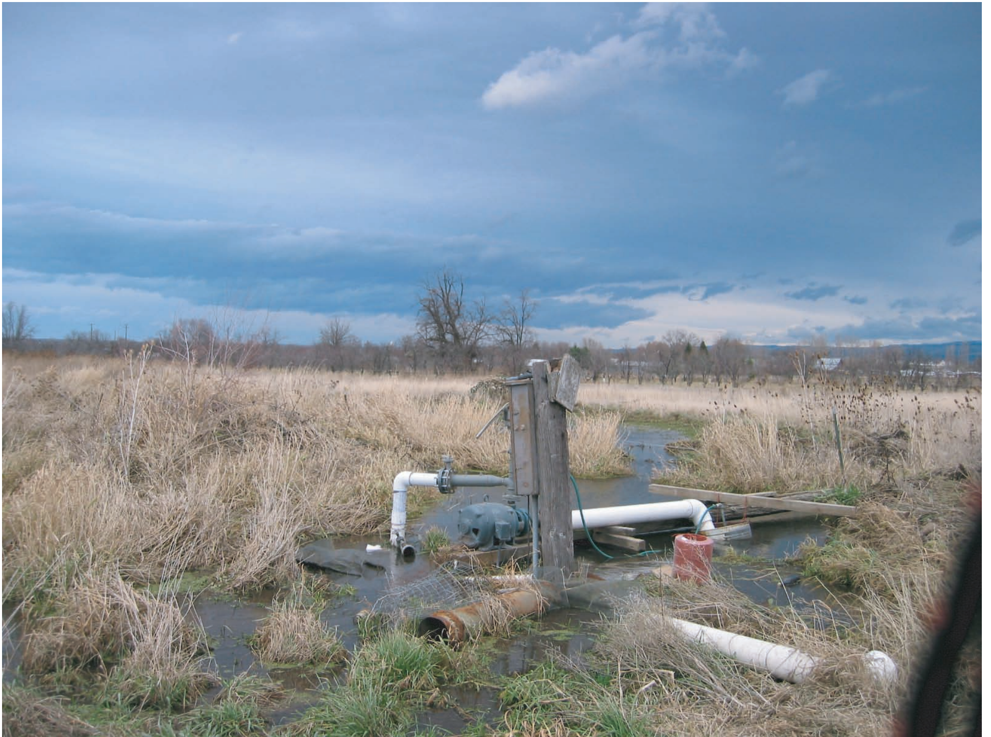
Figure 5. Irrigation pump sump pit at the Test Site
