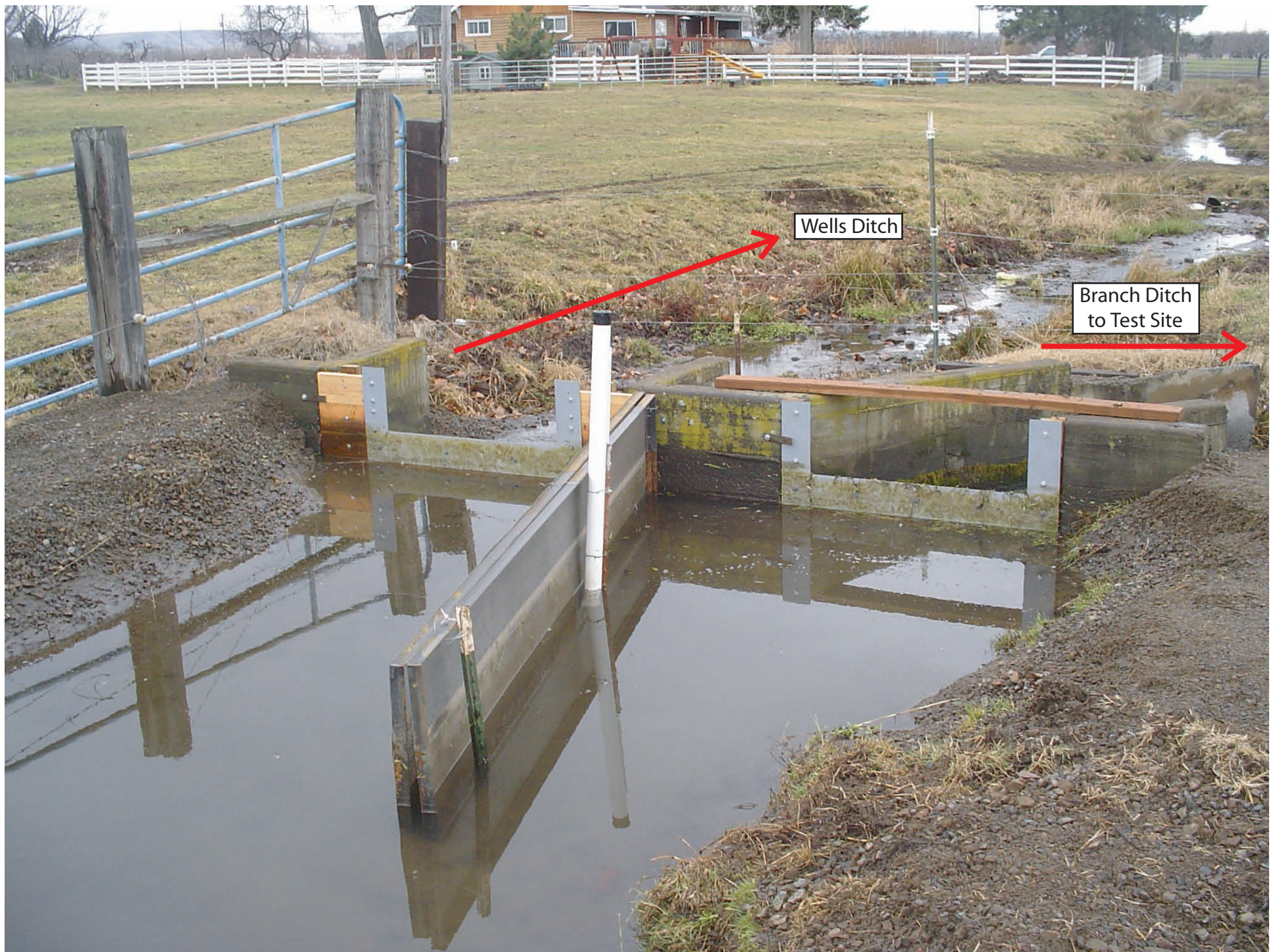
Figure 4. Photograph of the diversion head gate for the branch ditch on Wells Ditch.
