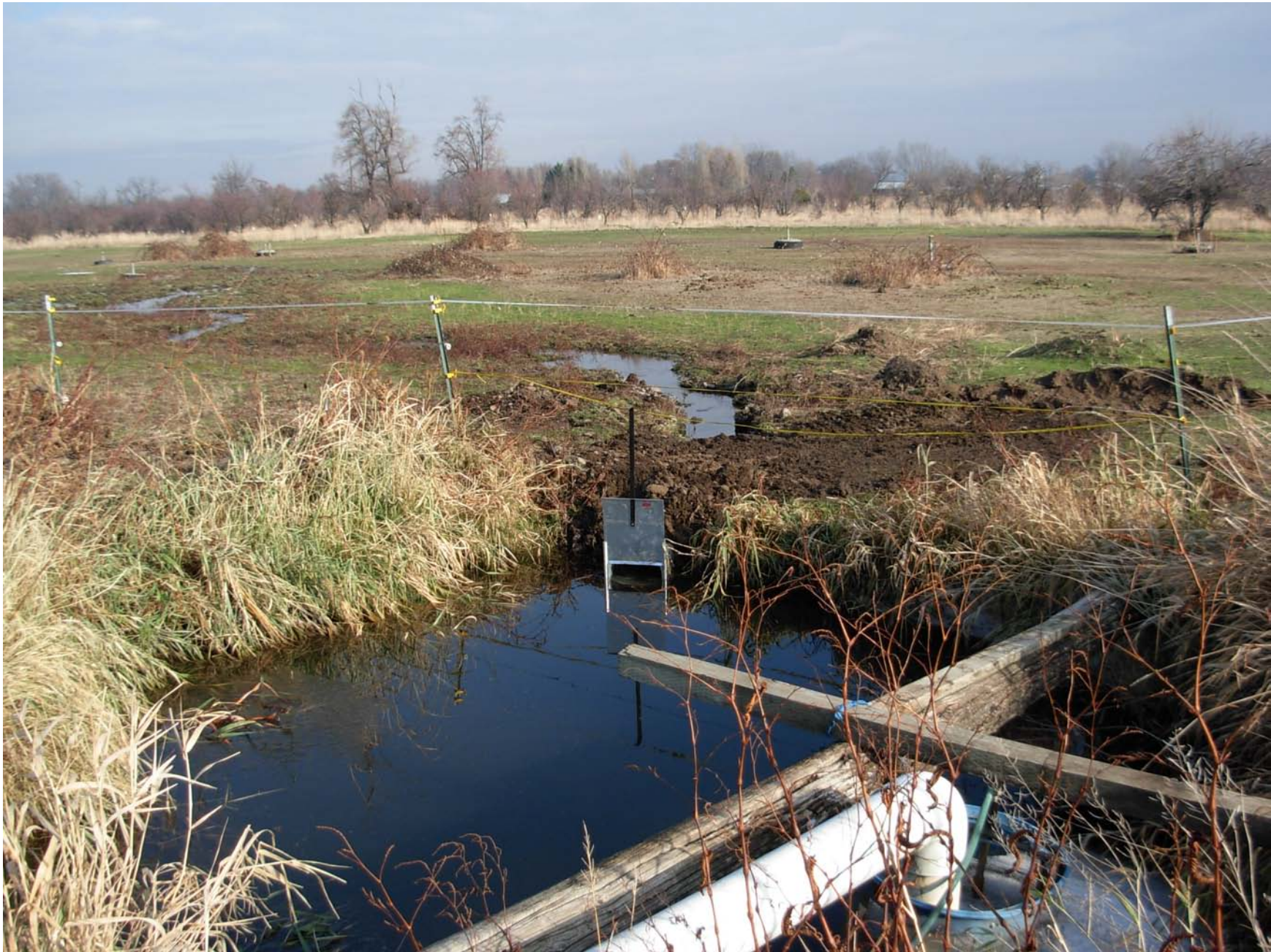
Figure 8. Photograph of the gated culvert used to control flow from the pump sump pit to the Hall portion of the Site.
