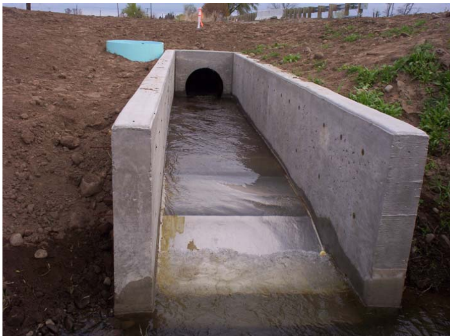
Figure 9. Head gate on the Gardena Farm Canal for the Locher Road SAR Site. View is looking to west-southwest, down stream on the Ditch. Site is just out of picture to the left.
