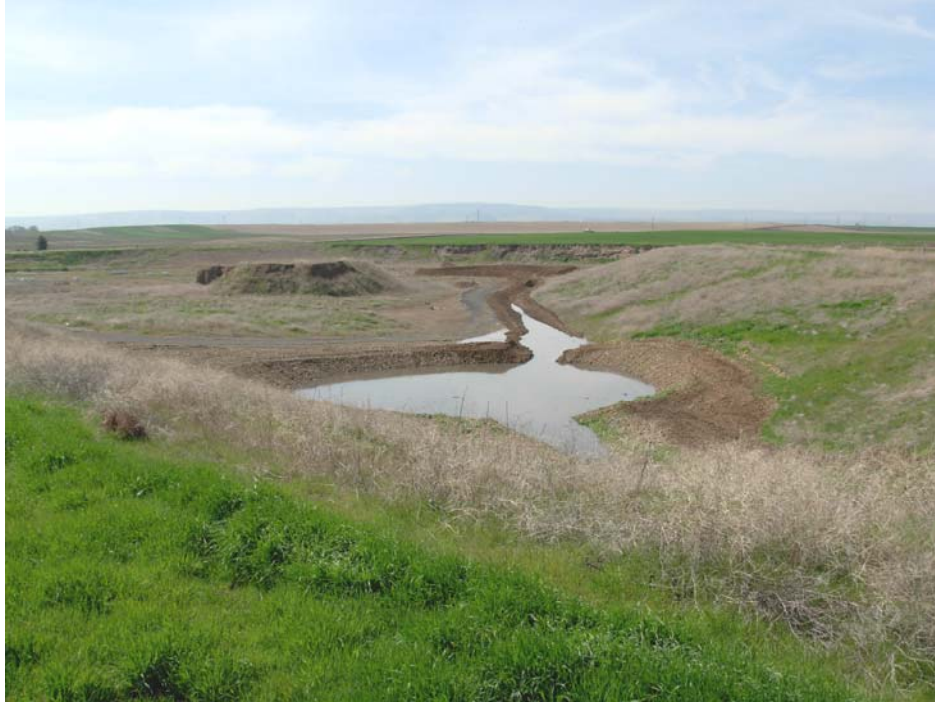
Figure 13. View to southwest looking across the upper basin and down the connector ditch leading to the lower basin, seen in the distance. Photograph was taken the first day the lower basin was used, 03 April 2007.
