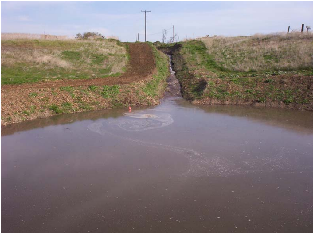
Figure 12. Upper basin as it was filling approximately mid-test.
