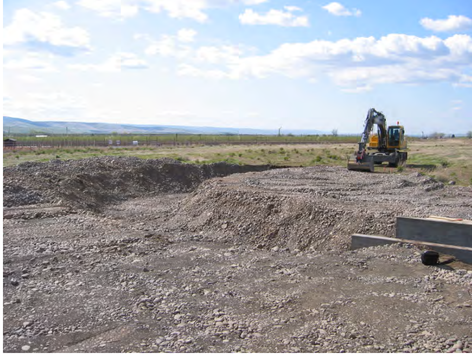
Figure 11. Photograph of gray colored excavated gravel of the Quaternary coarse unit. This trench was dug at the WWBWC/Hudson Bay SAR Site.
