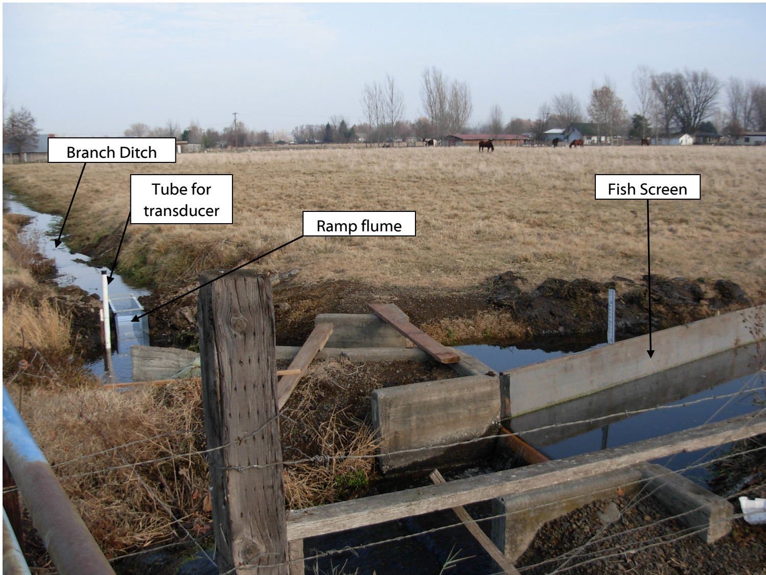
Figure 4. Ramp flume at upstream end of Branch Ditch. The vertical white tube is where the transducer is installed. The Wells Ditch fish screen and diversion weir is in the foreground. This view is to the north.
