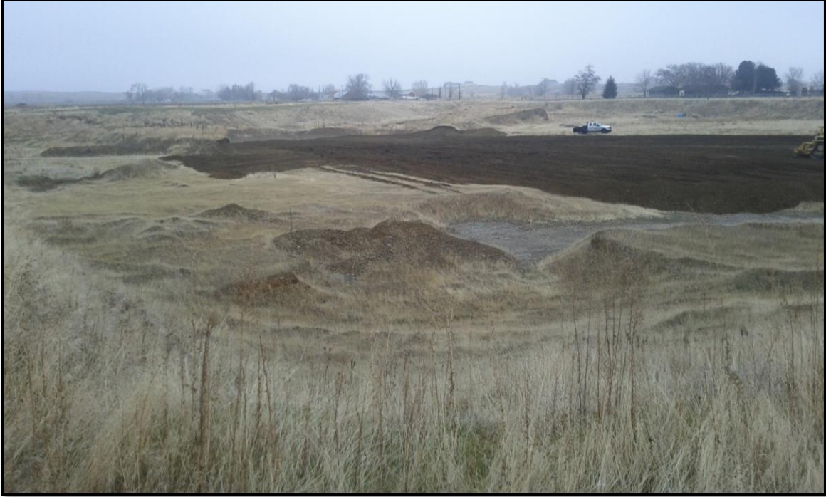
Figure 12 - Photo during expansion of the Locher Road site's main recharge basin, December 2011.
