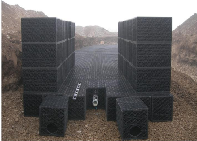
Raintanks being deployed
