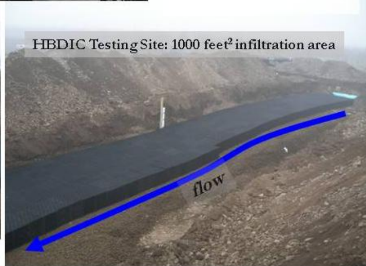
Figure 60. Infiltration Gallery #4 - Atlantis Raintanks Installation (2008)
