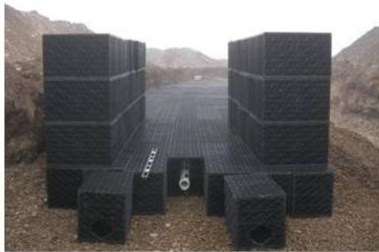
Raintanks being deployed
