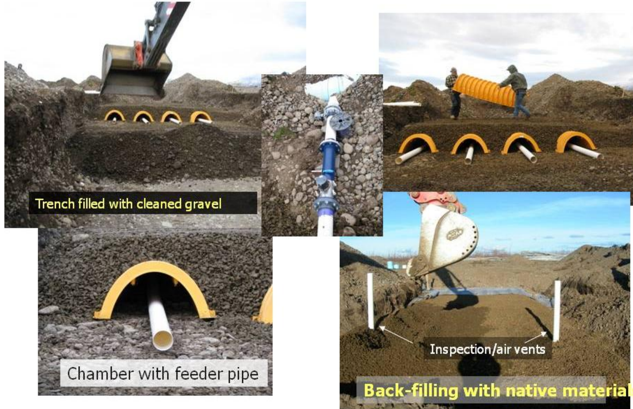
Figure 59. Infiltration Gallery #3 - Stormtech Chamber Installation (2008)
