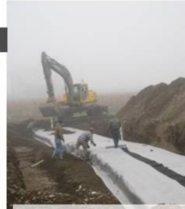
Gallery top: filter fabric and mesh
