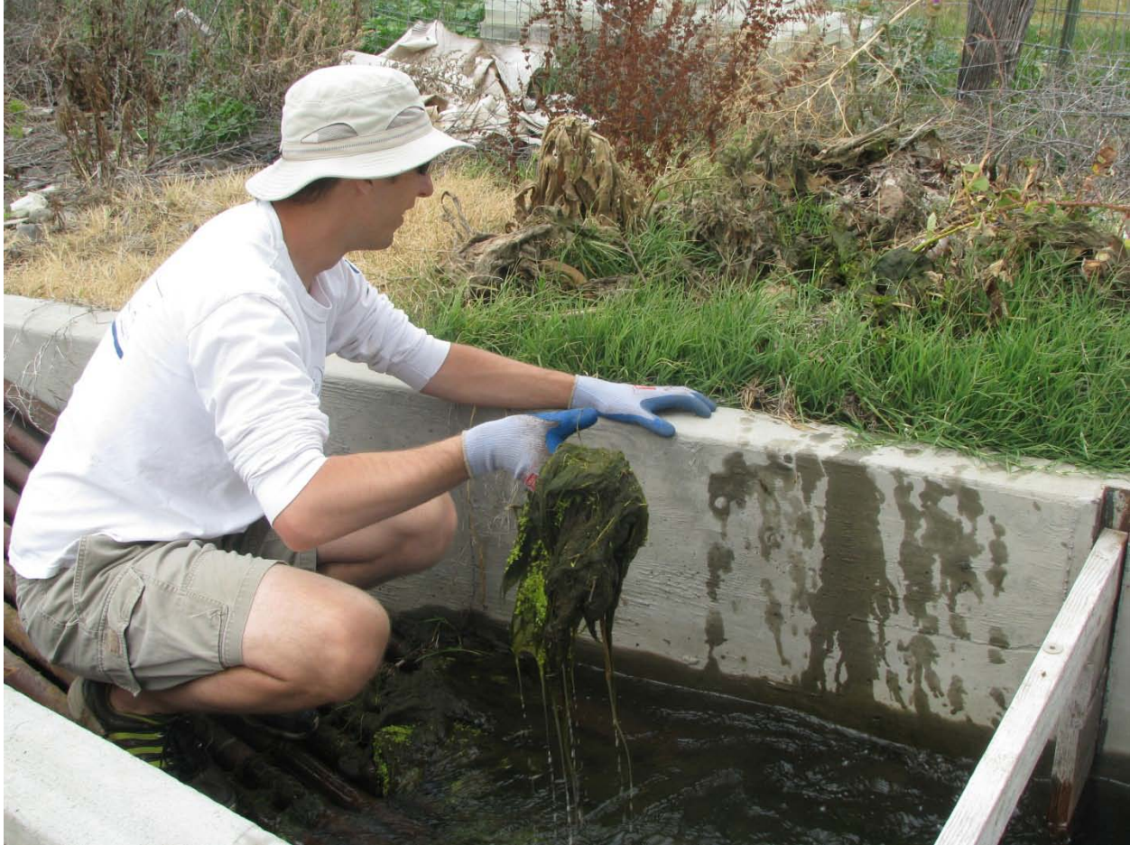
Figure 15. S-410, Johnson Creek in Umapine, now has trouble with pond algae clogging the grating.
