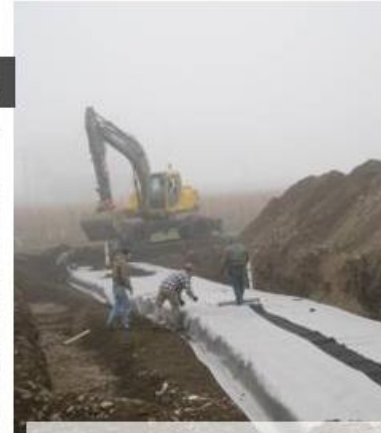
Gallery top: filter fabric and mesh
