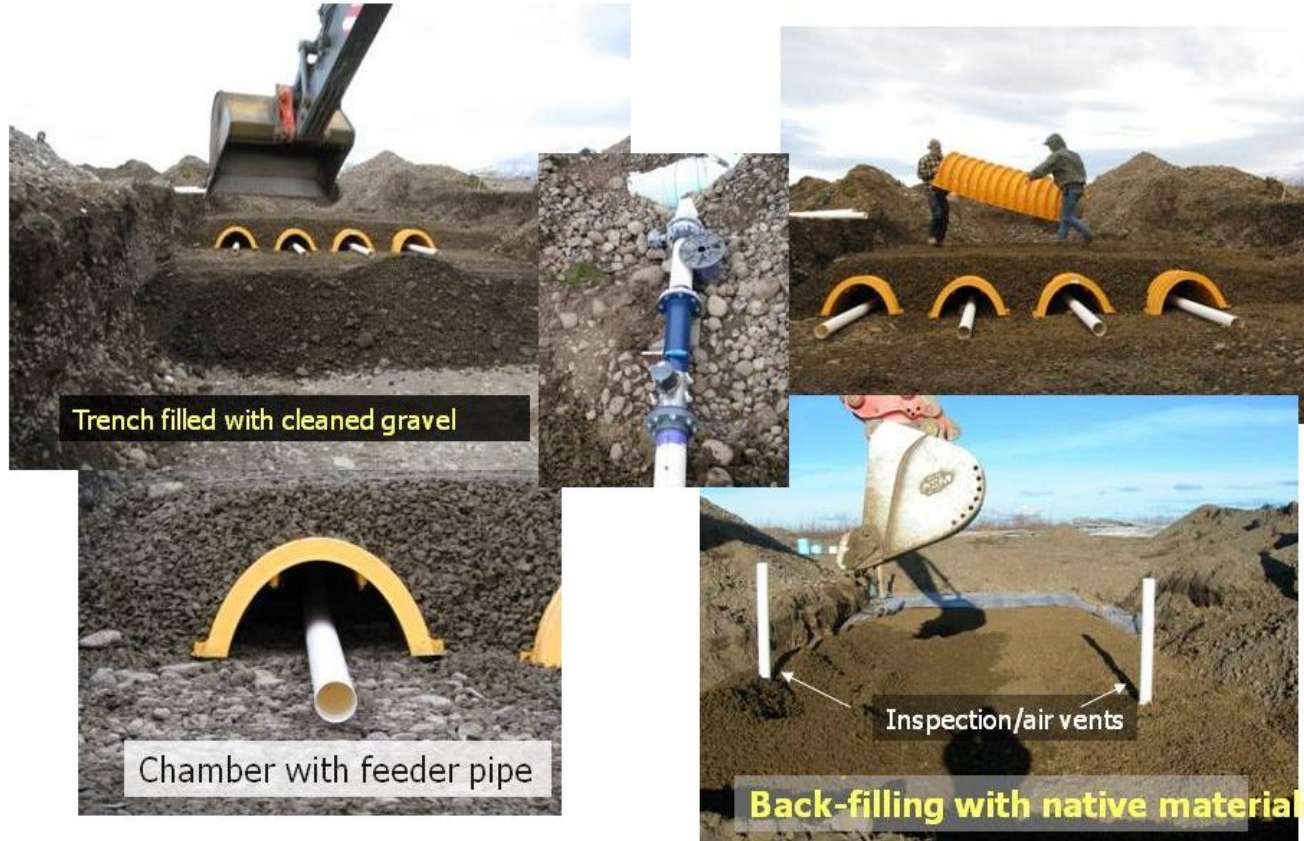
Figure 59. Infiltration Gallery #3 - Stormtech Chamber Installation (2008)
