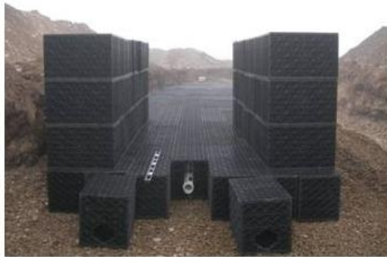
Raintanks being deployed
