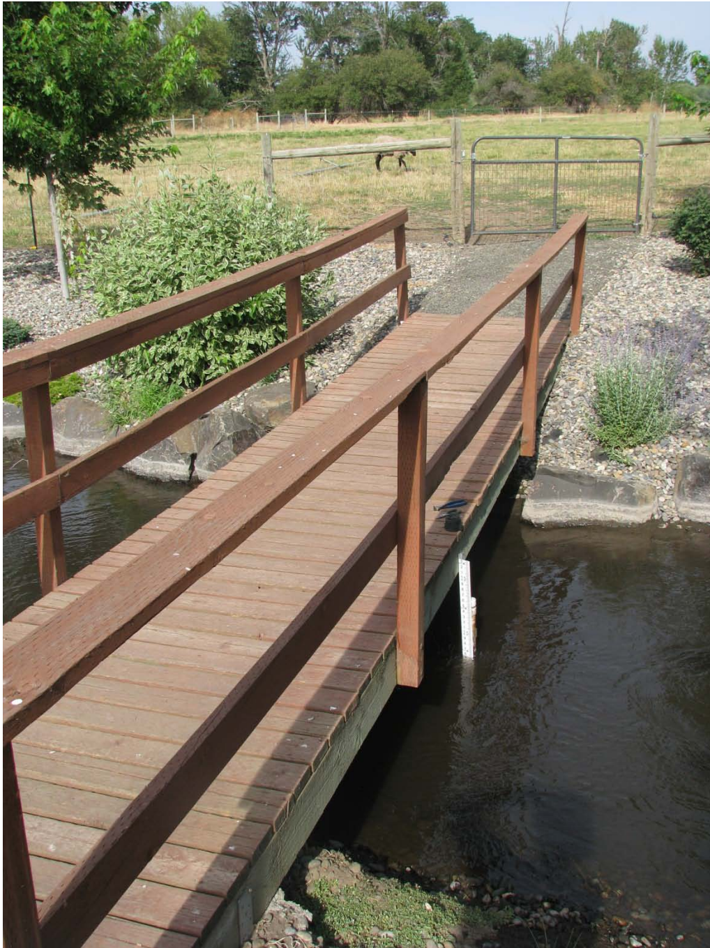
Figure 5. This is the new location for the S226 gauge on the East Little Walla Walla River. Typical of many WWBWC gauges, a PVC stilling well and a staff gauge are lashed to a fence post imbedded in the channel.
