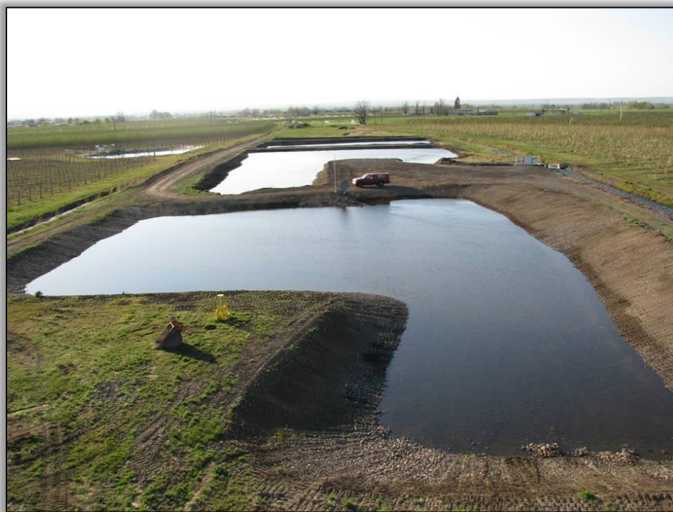
HBDIC Recharge Project Expansion with Basin #1 (foreground), spring 2008
