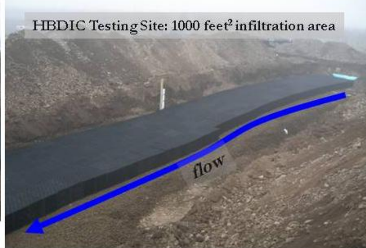
Figure 60. Infiltration Gallery #4 - Atlantis Raintanks Installation (2008)
