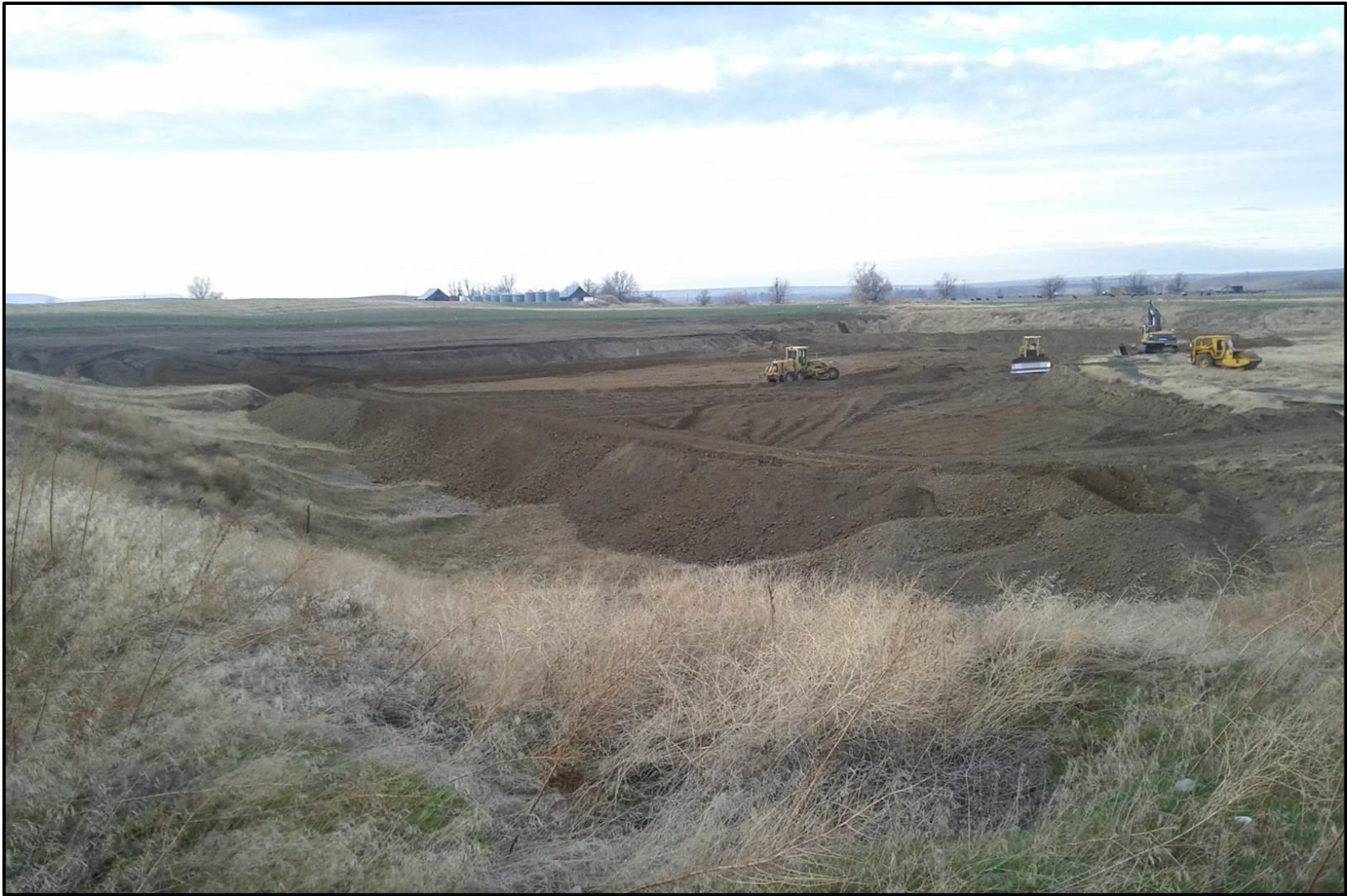
Figure 5- The Locher Road Aquifer Recharge Project during expansion activities in late 2011. The project was expanded from ~1/3 acre basin to a ~2 acre basin. The project basin is located within a historic gravel quarry.
