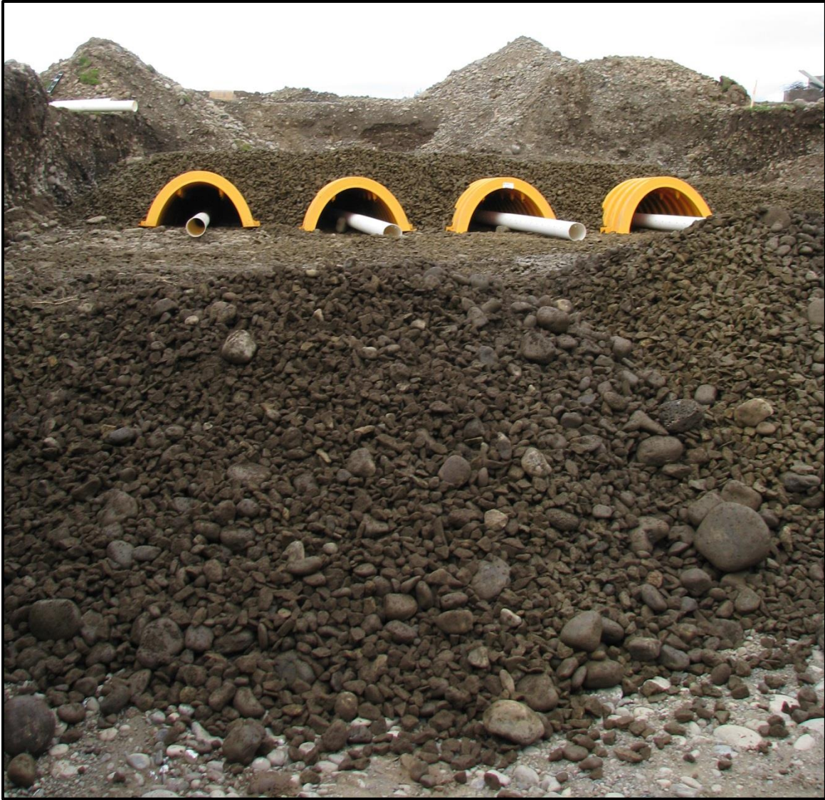
Figure 13 - Photograph of infiltration gallery #3 (IG3) at the Johnson Aquifer Recharge site. IG3 is 4" perforated drain field pipe installed within Stormtech stormwater chambers (yellow covers) over washed gravel and buried in ~2 foot of washed gravel with geo-textile fabric on top of the gravel. See Appendix D for designs.
