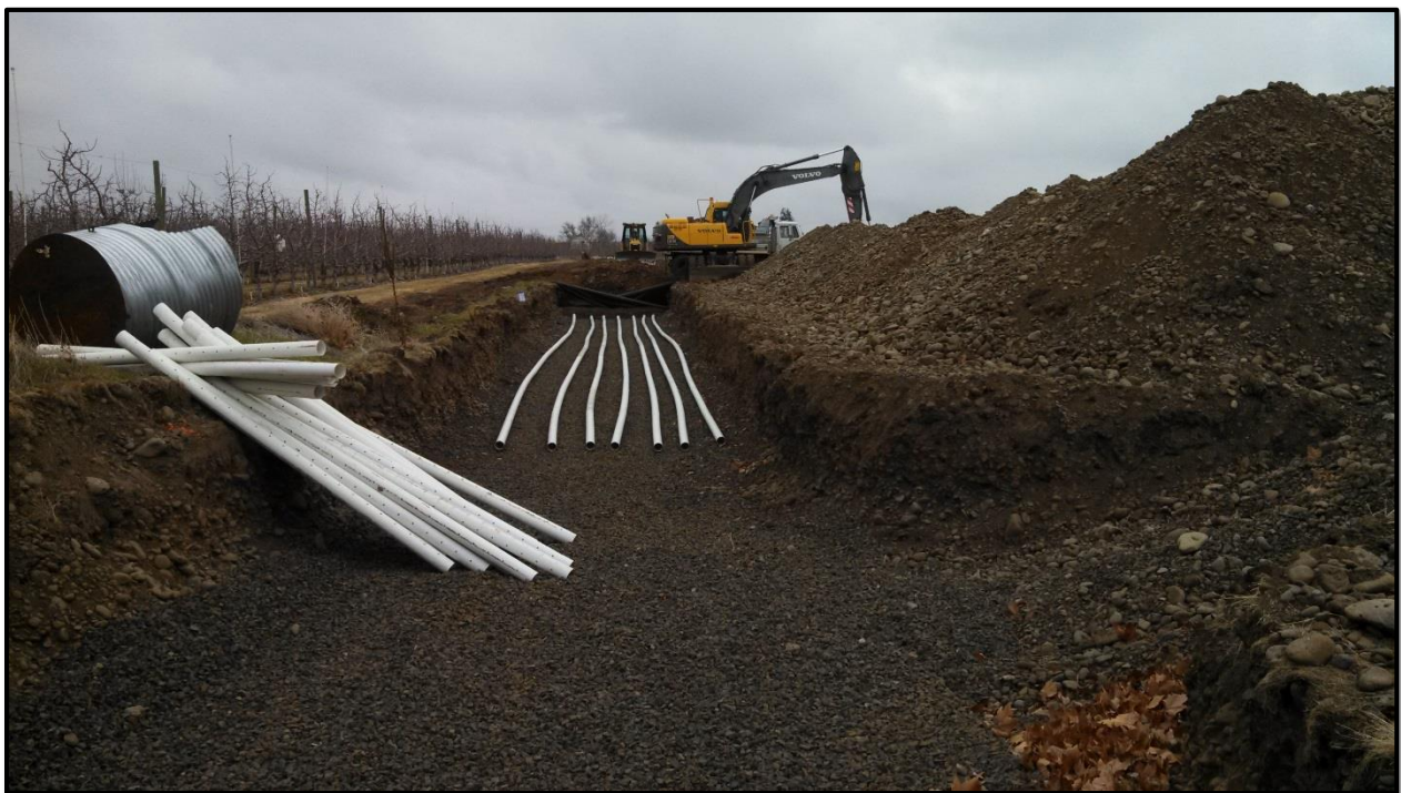
Figure 12 - The Barrett Aquifer Recharge site during construction in January 2014. This recharge site utilizes 7 4-inch perforated pipes that run approximately 600 feet. See Appendix C for designs.
