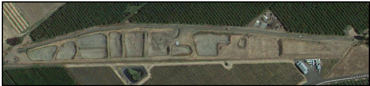
Figure 15 - Aerial photo of the Johnson site from 2013 showing the current configuration of the site with 10 spreading basins and 3 active infiltration galleries (between the spreading basins and the pile of fill material).
