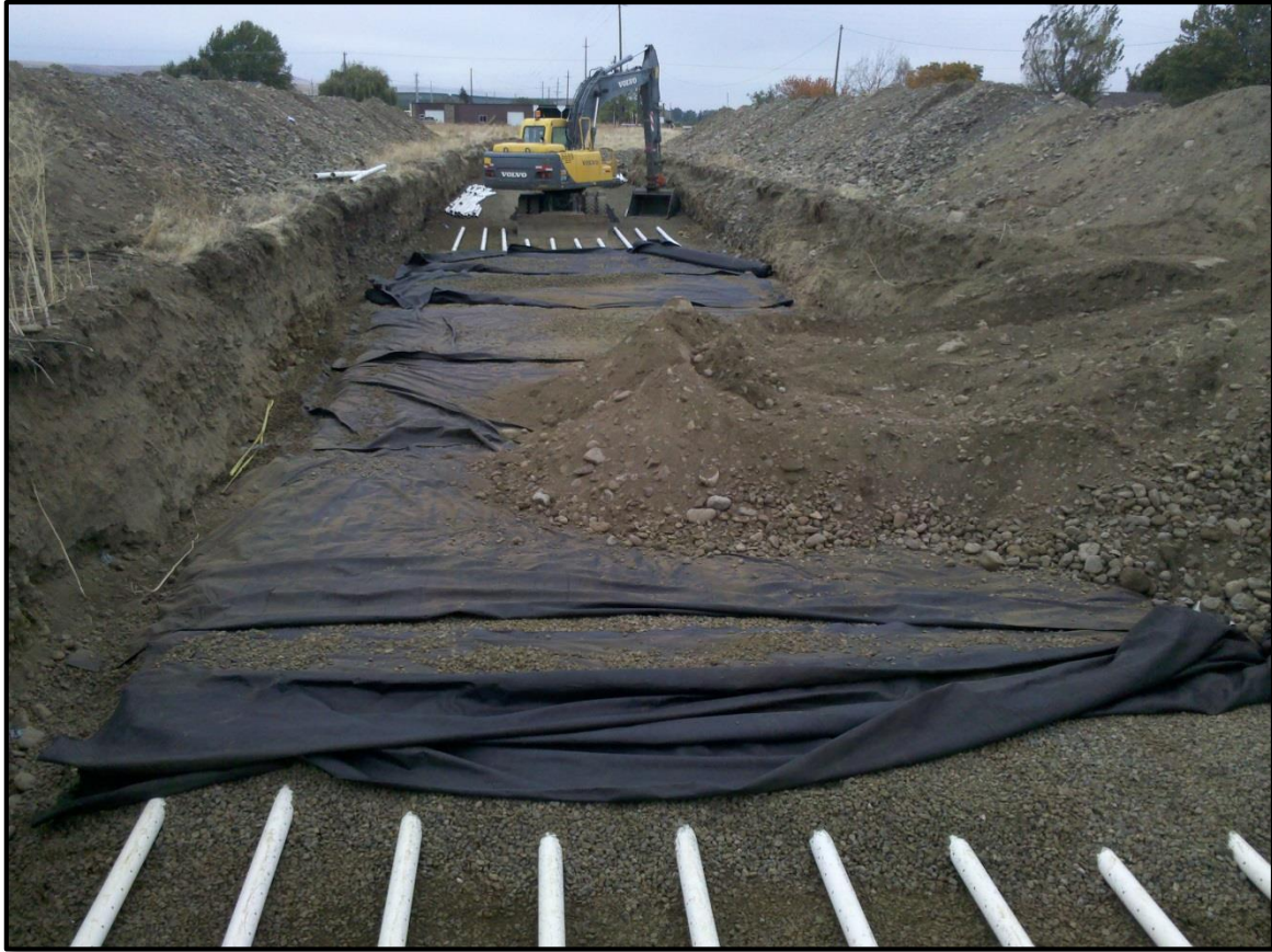
Figure 10 - The Anspach Aquifer Recharge site during construction in October 2012. This recharge site utilizes 10 4-inch perforated pipes that run approximately 200 feet. See Appendix C for designs.
