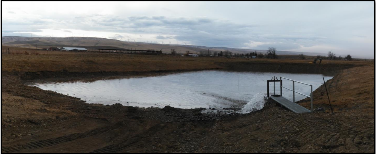
Figure 20 - NW Umapine Aquifer Recharge site operating during the WY2014 recharge season.
