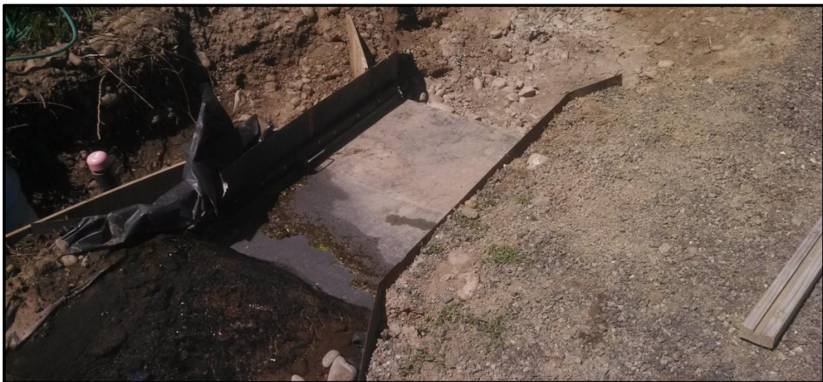
Figure 10 - The Anspach Aquifer Recharge site during construction in October 2012. This recharge site utilizes 10 4-inch perforated pipes that run approximately 200 feet. See Appendix C for designs.
