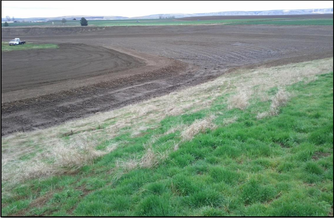
Figure 13 - Photo of the completed expansion of the Locher Road site's main recharge basin, December 2011.
