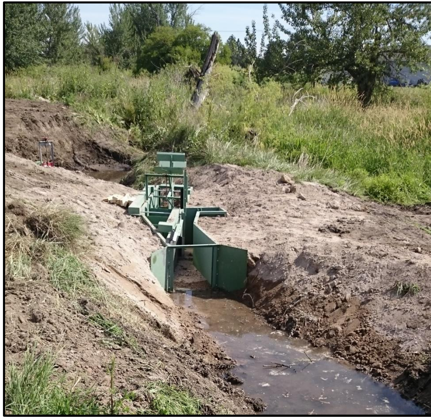
Figure 18 - Irrigation ditch, fish screen and intake (back left) for the Last Chance Road Aquifer Recharge site.
