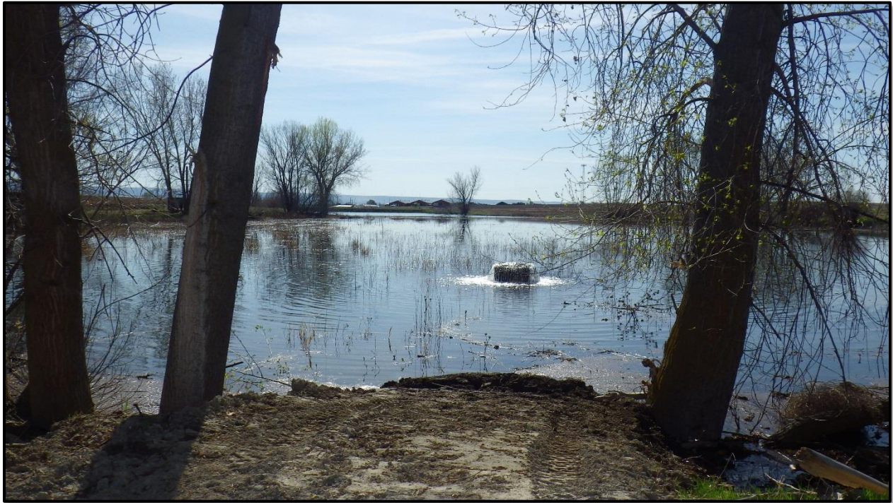
Figure 16 - Stiller Pond Aquifer Recharge site during operations.
