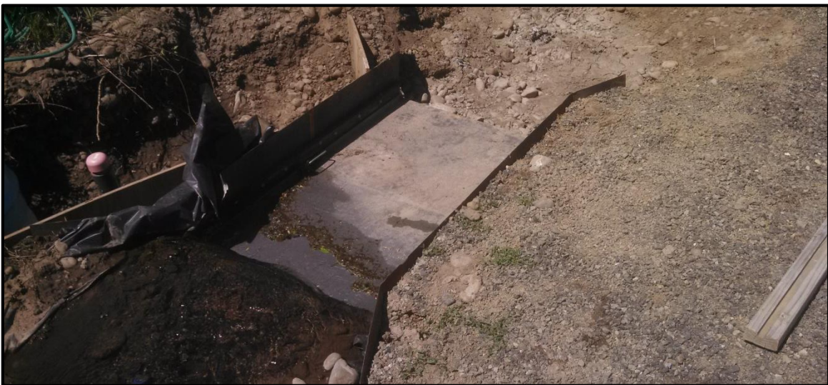
Figure 11 - The turnout structure for the Anspach Aquifer Recharge site.
