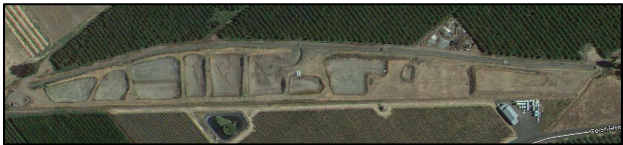
Figure 15 - Aerial photo of the Johnson site from 2013 showing the current configuration of the site with 10 spreading basins and 3 active infiltration galleries (between the spreading basins and the pile of fill material).
