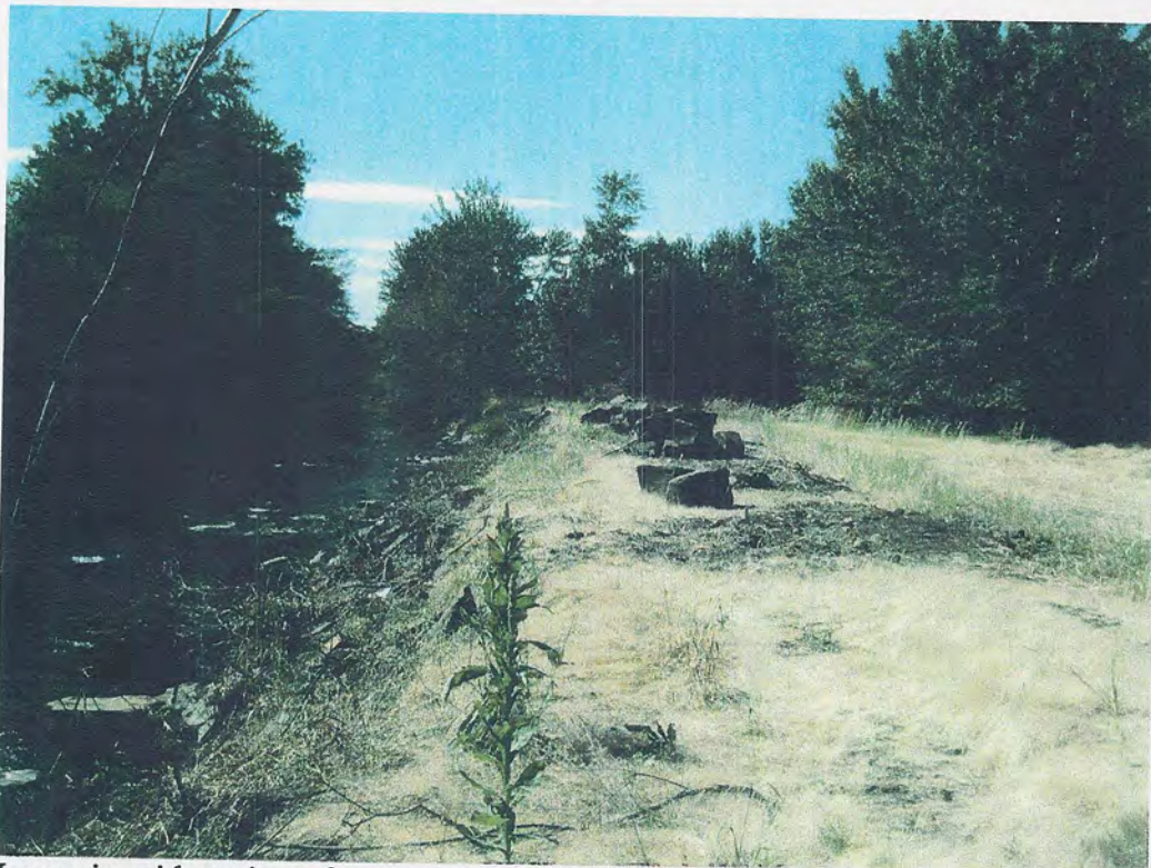
Levee in mid section of project prior to removal
