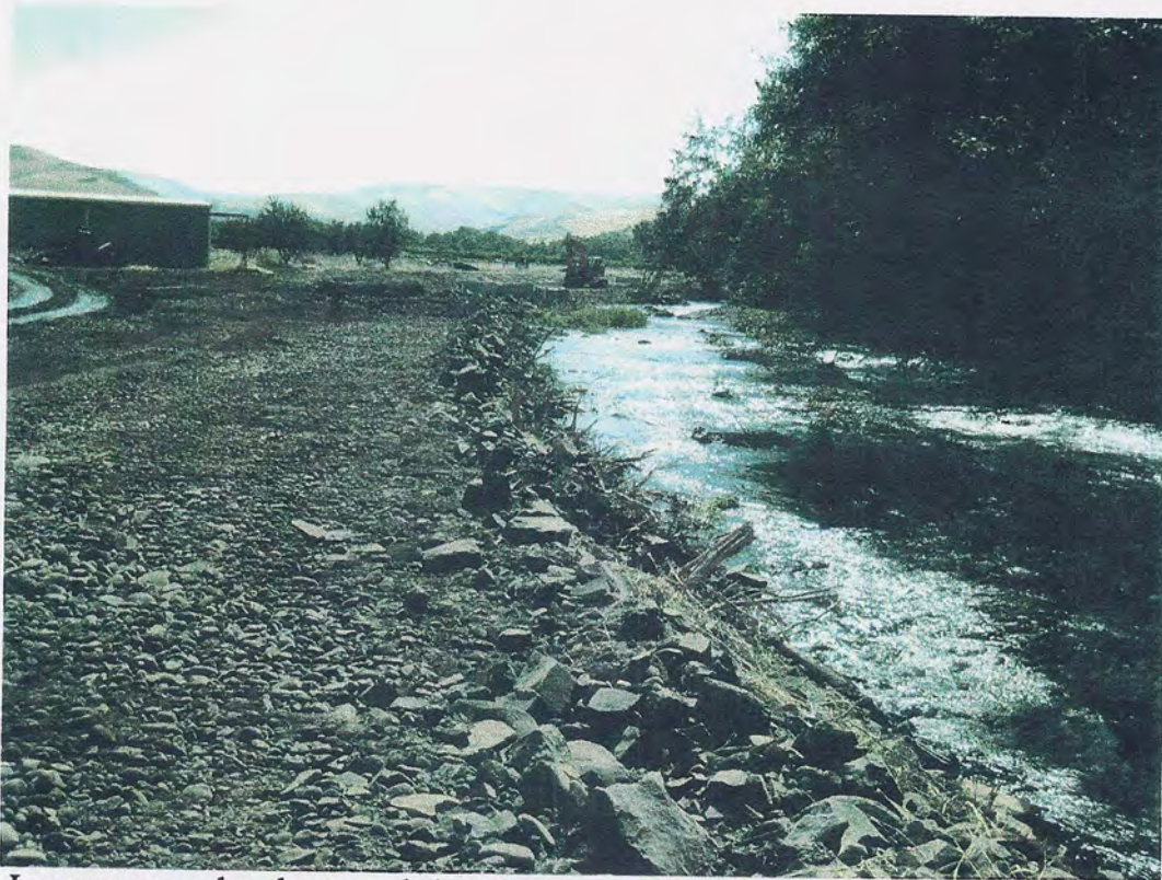
Levee removed and rootwads installed
