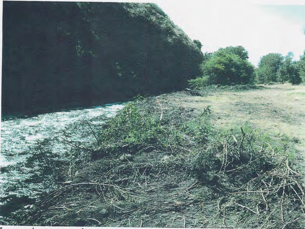
Levee prior to removal
