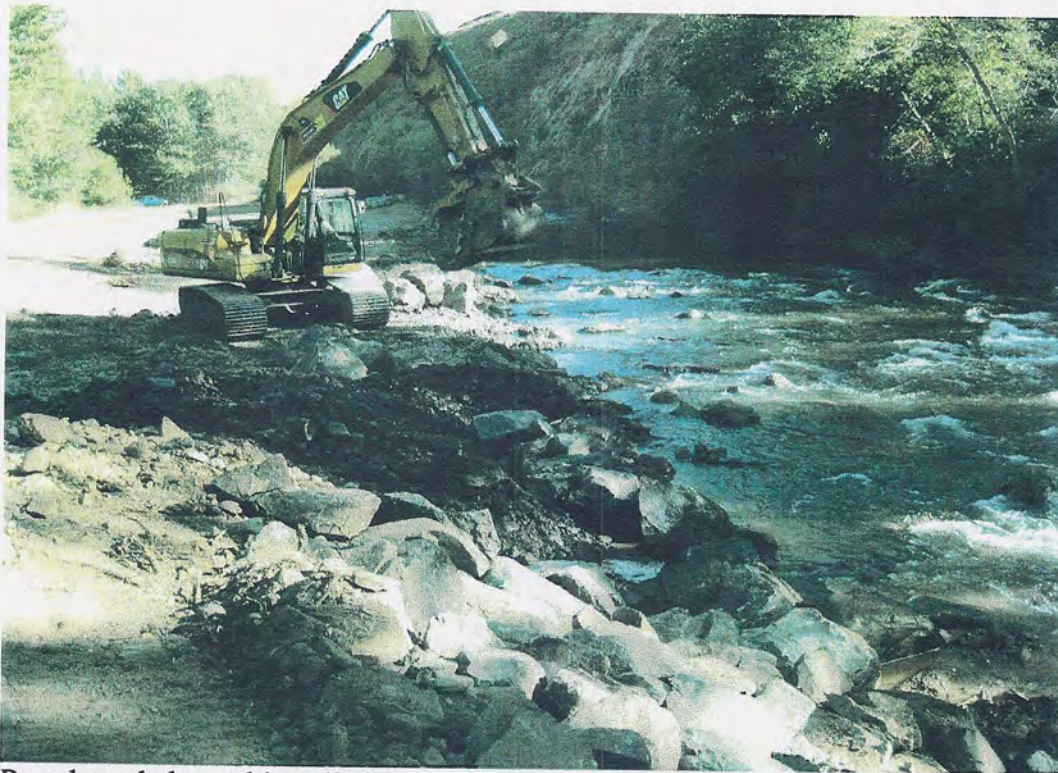
Roughened channel installed at downstream end of project to maintain grade
