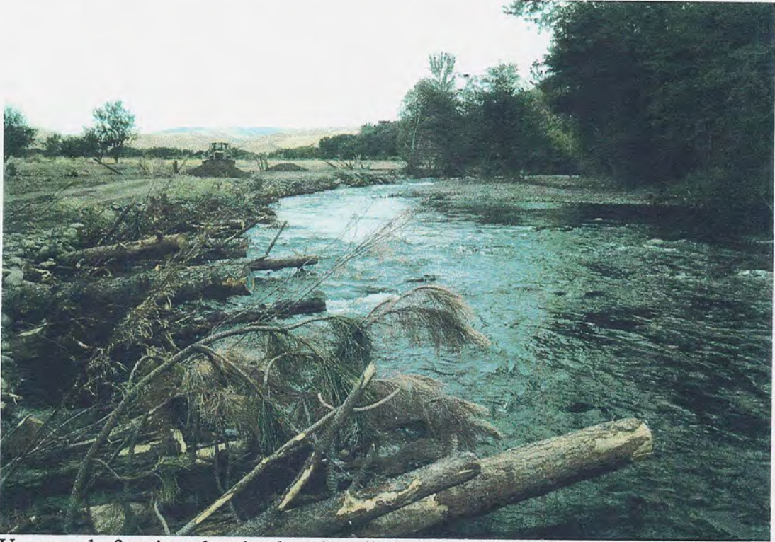
Upper end of project showing logs installed and habitat rocks
