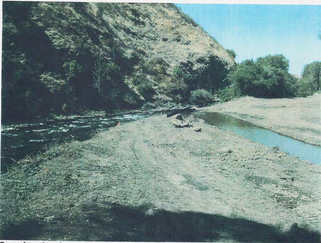
Same location, levee gone and side channel being installed
