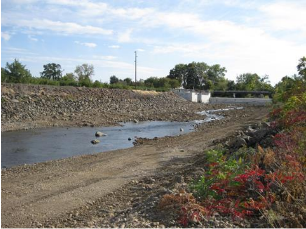
Project photo immediately after project completion
