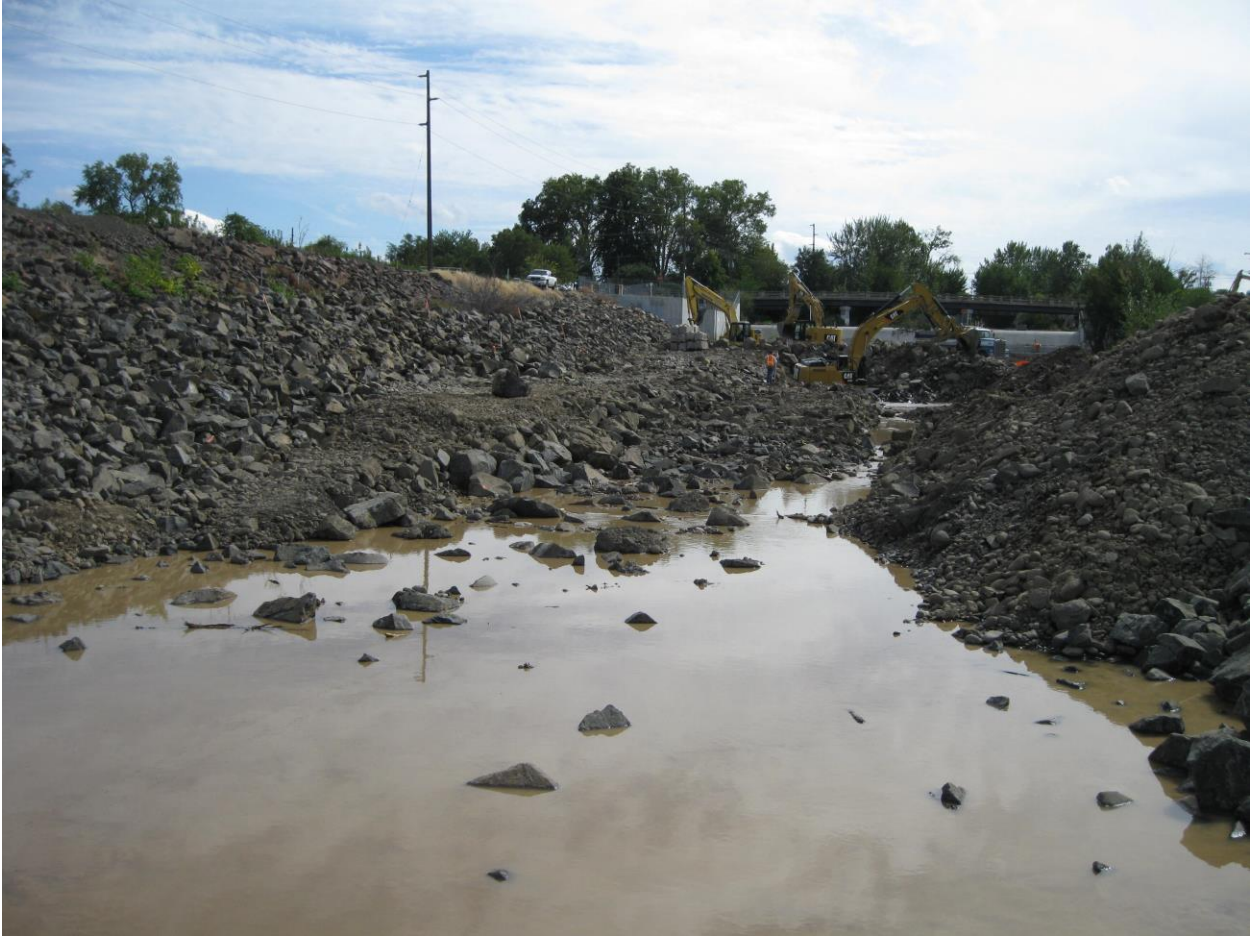
Project site during construction
