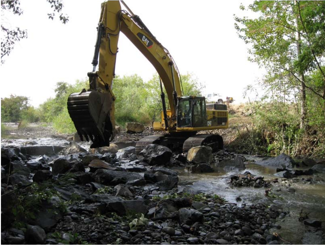
This photo shows Partney Construction's operator building the roughened channel.
