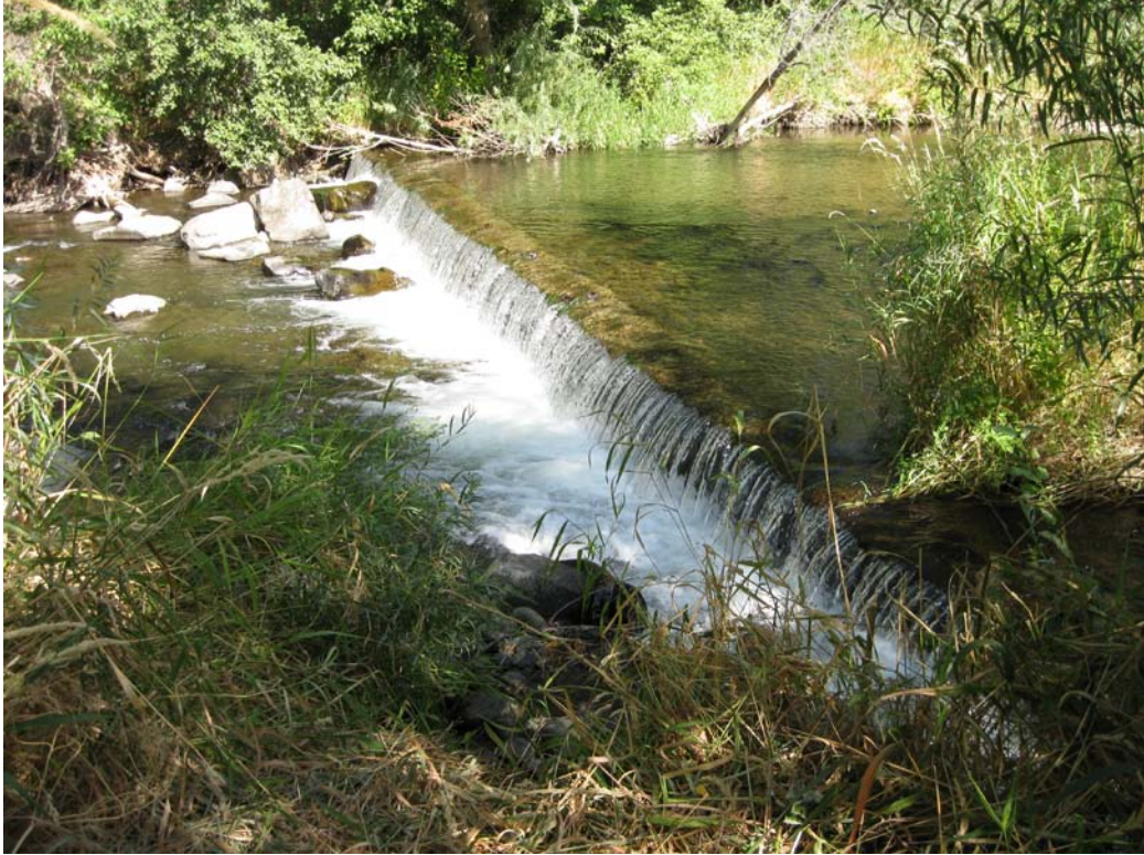
This pre-construction photo shows the fish passage barrier created by the Walla Walla river stream bed downcutting downstream of the Corps of Engineers' concrete grade control structure. The concrete structure was installed the late 1940s.
