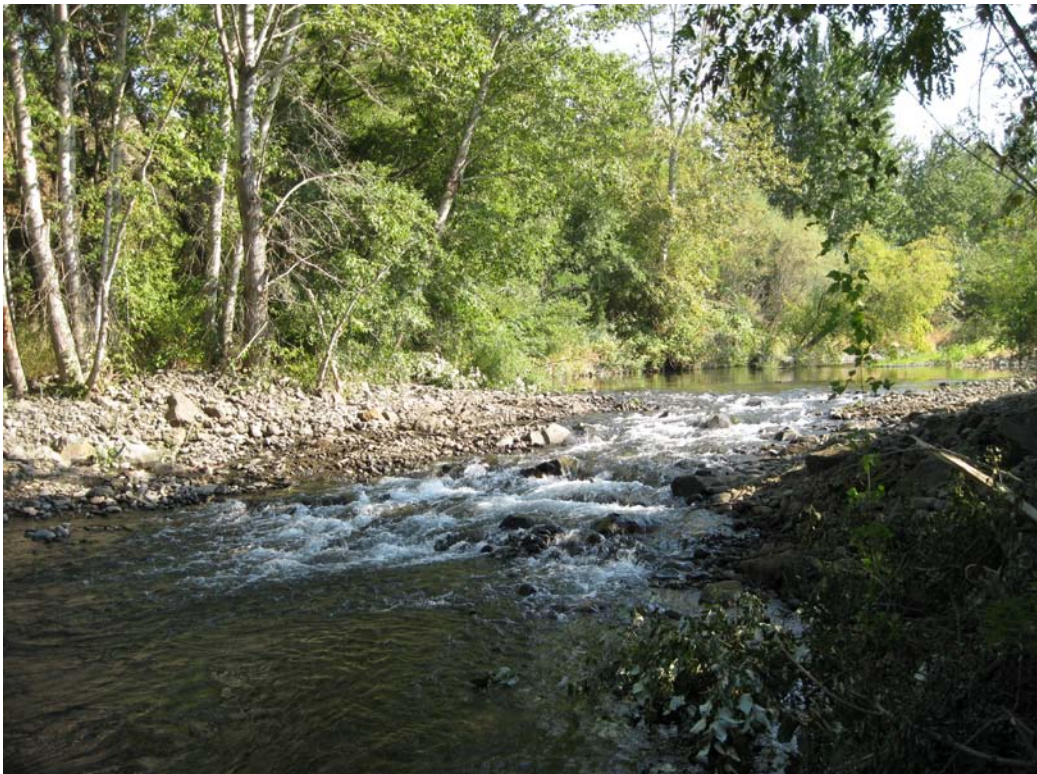
This photo shows the completed project. Rock has been placed downstream of the notched concrete to maintain a sloped channel that fish can negotiate.
